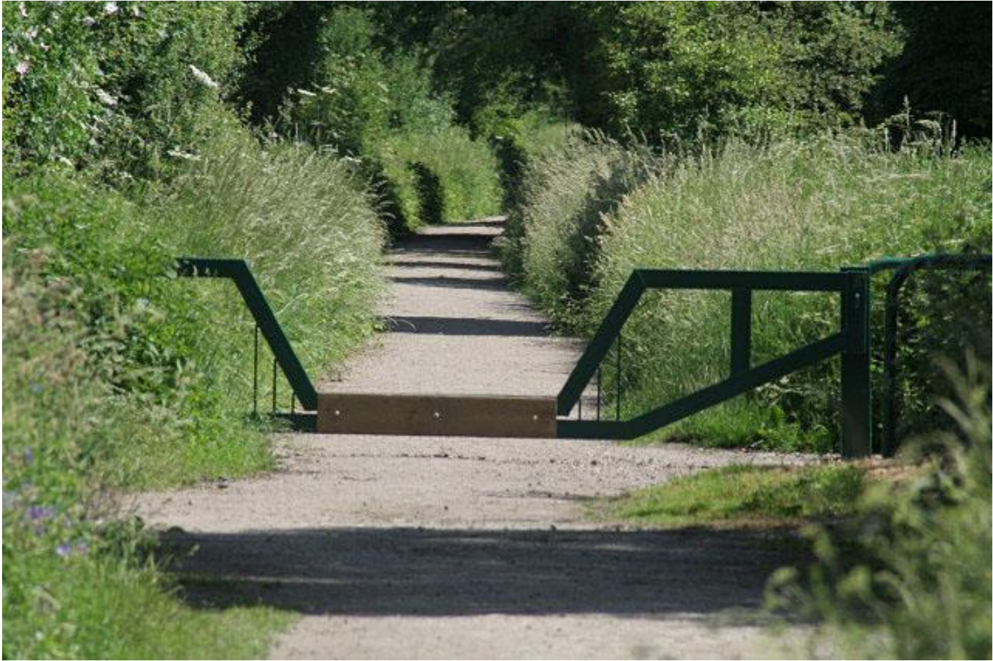
Infrastructure Barriers - Horse Stiles
